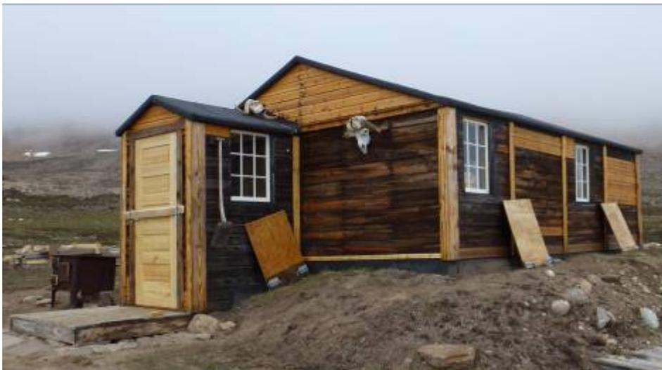
*Dødemandsbugten at our departure. The house is now fully renovated with a new door and new windows. It was a conscious choice to keep the fine, rustic board facade and to exchange only the rotten boards.*
